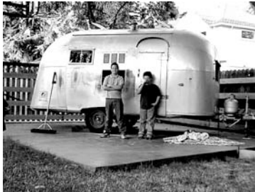
After demolition with Mike and Eric
