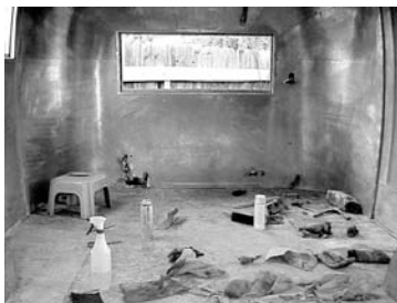
7 layers of paint removed
