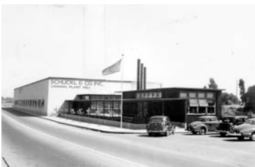
Schuckl Plant No. 1, 1944, Photo Courtesy of Environmental Design Archives, WBE Collection, UC Berkeley.
