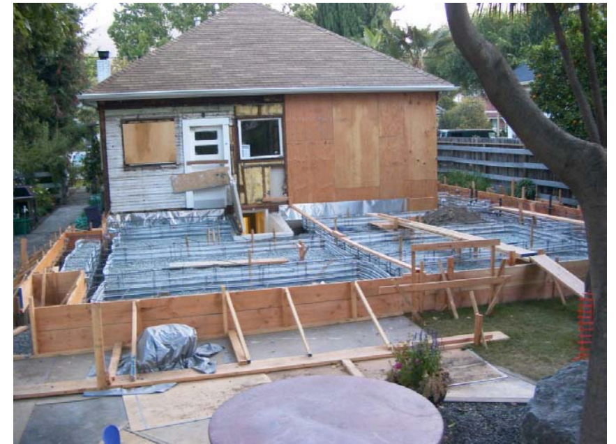
This photo illustrated the build-up of the grade beam grid and Slab.
