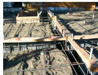
Sand over Vapor barrier over crushed rock prior to concrete pour
