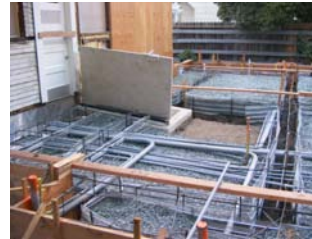
Build up of grade beam grid & slab Detail
