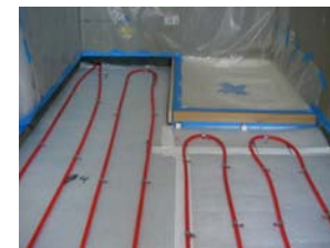
Radiant Installation
