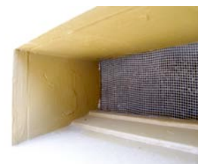
Pest & Bug screen at 1910 House Cellar vents
