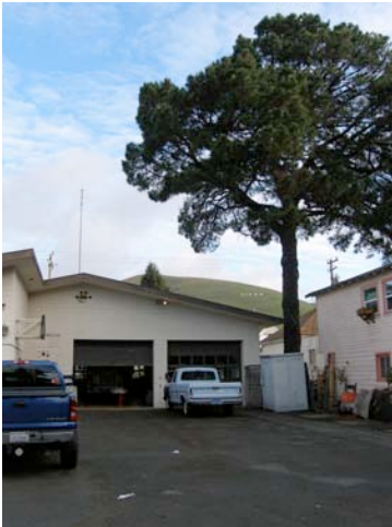
The City paved the alley behind the Fire Station, but did not have to prove they had the legal right. Commercial Alley, 2006.
