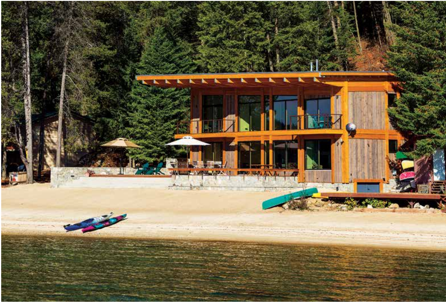
ABOVE: Glue laminated timbers, commonly known as glulams, add architectural interest to the home's overhang and are ideal for carrying the extra weight of heavy snow loads.
